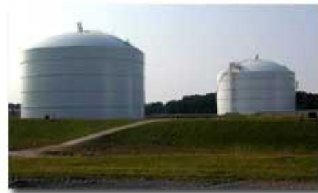
LNG Storage Tanks Cove Point Import Terminal, Maryland Photo courtesy of Dominion © 2003, www.dom.com
